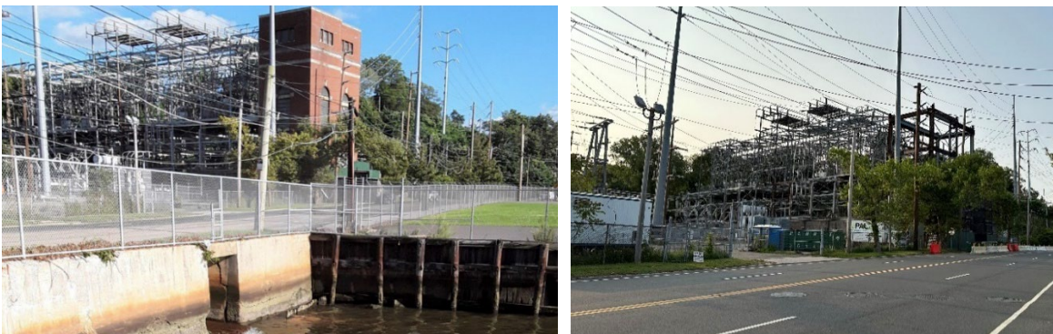
CSHH #14A, powerhouse drain outfall (l) adjacent to the lot that was the site of the old brick powerhouse building; post-demolition of brick structure (r) on east side of the road (photos by Carol DiPaolo, 9/2/21, and Michelle Lapinel McAllister, 5/24/23, respectively)
