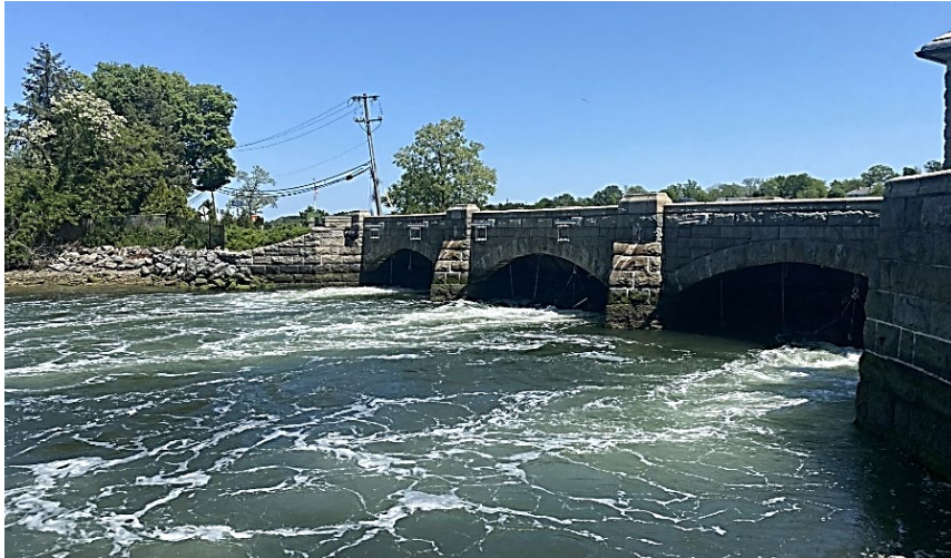
Tidal gates north of the bridge on the west side of Dosoris Pond, station “DP3” (photo by Evelyn Powers, 5/17/23)
